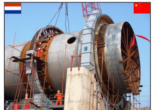
Installing the girth gear, manufactured in the **Netherlands**, onto the outer shell.
