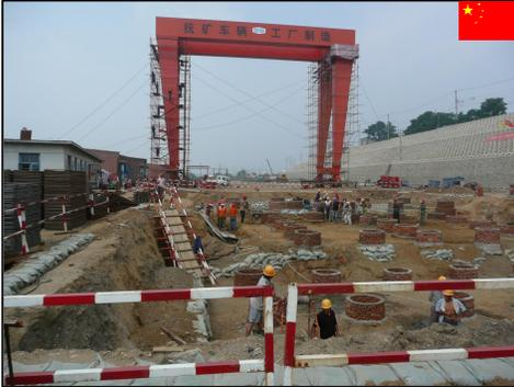
View of the site for the ATP System plant, showing preparations for installation of concrete pile. The pile excavations were dug by hand! The gantry crane extends the length of site for use during construction.
