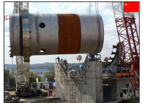
Lifting one section of the ATP Processor outer shell and one support tyre onto the foundation. Balloons and fireworks were provided by FMG to celebrate this achievement.
