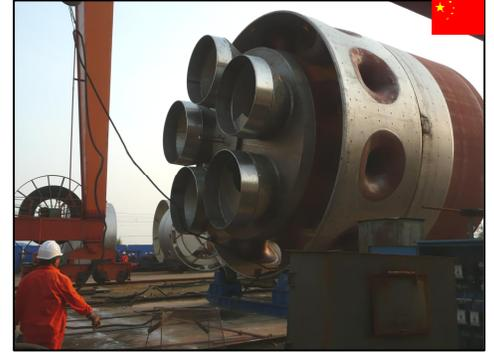
Field welding of the centre support section in **China**. A total of fourteen 8.5 m diameter circumferential welds in steel up to 100 mm thick were required to join 15 outer shell segments together.
