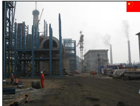
View of ATP Plant showing control room on right hand side and steel platforms being erected.
